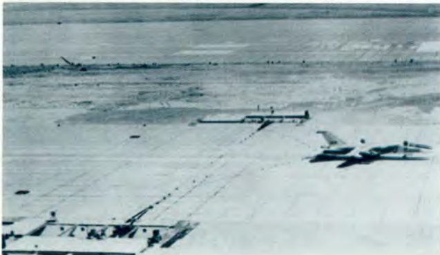
F-111 engages BAK 12 during tests in the early '60s.
